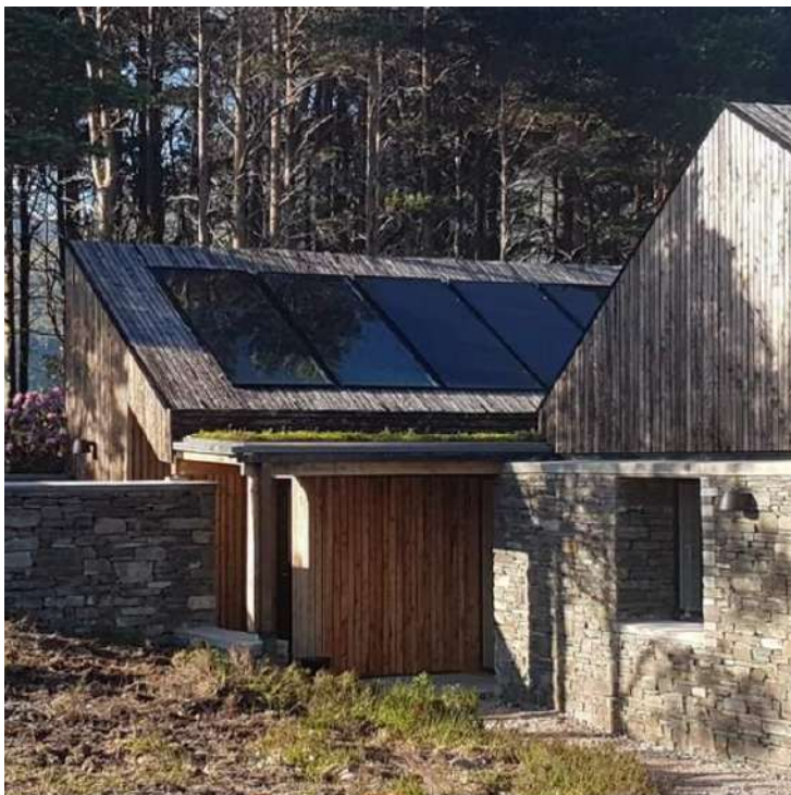
Solar panels at off-grid Lochside House by Haysom Ward Millar, Scotland
