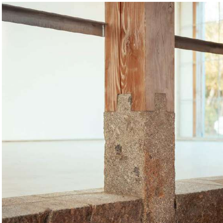
Stone to timber connection by Thomas Randall Page, Art Barn, Devon
