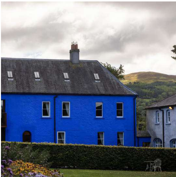
School House by Canice Architects, County Tipperary, Ireland
