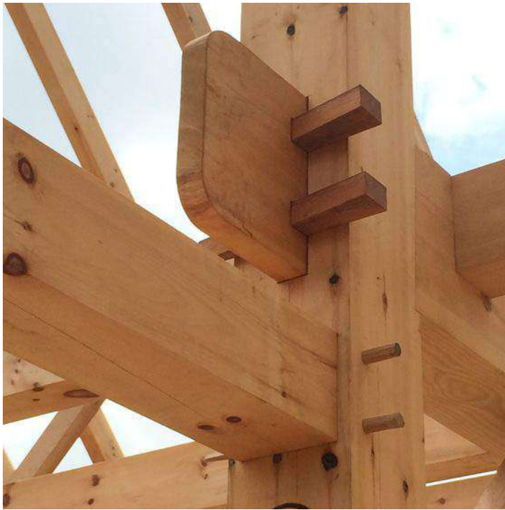
Dry-fit all-timber connections made with pegs
