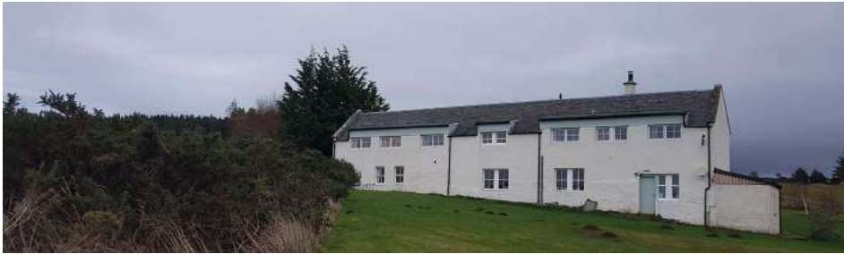
West elevation of main building
