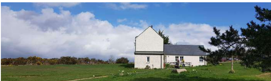
South gable of main building with kitchen and office extension wing at right
