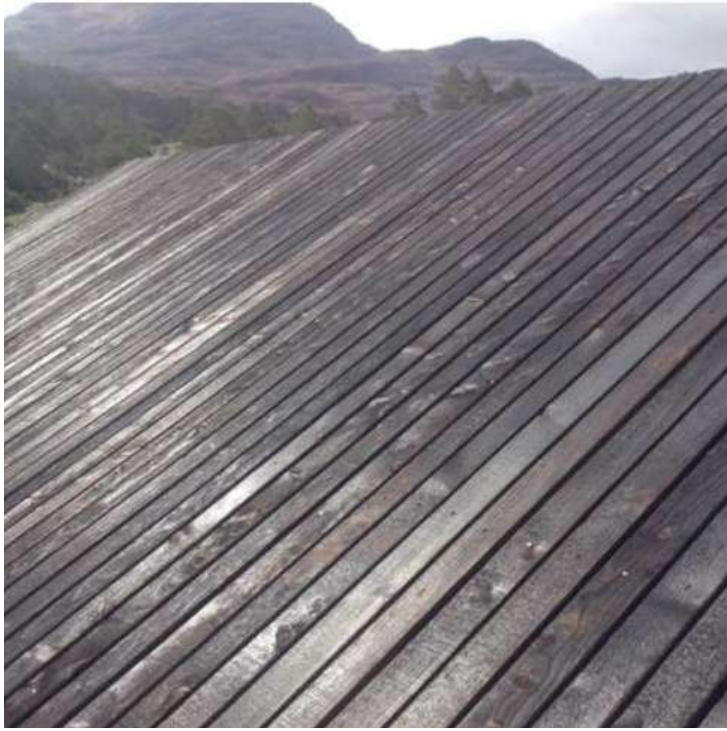
Timber roofing at Lochside House by Haysom Ward Millar, Scotland
