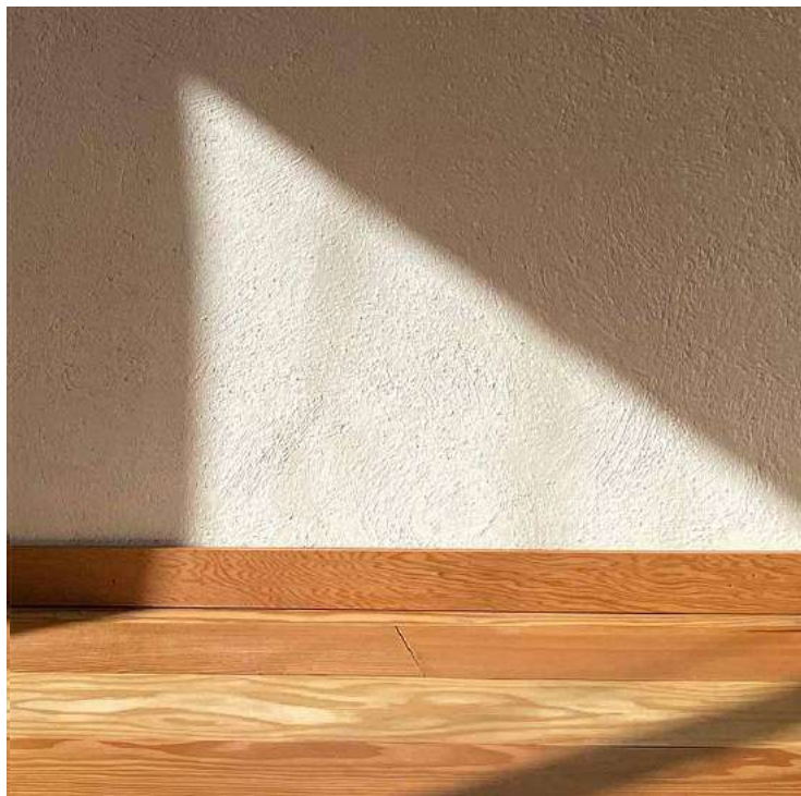
Lime-hemp plaster, The Lighthouse by Taigh Solais Architecture, Edinburgh
