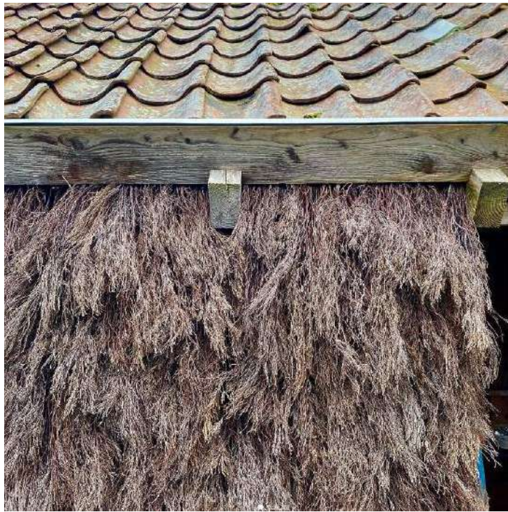
Traditional heather thatch used on a wall, photo by Becky Little, Scotland
