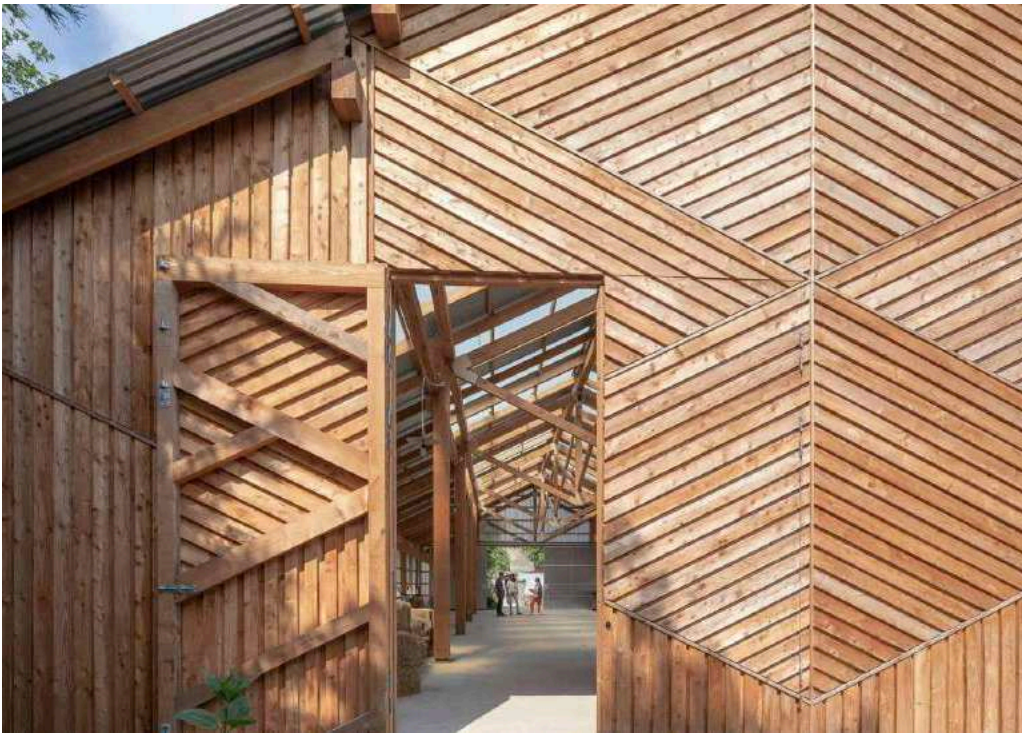
Timber cladding patterns, Waterloo City Farm by Feilden Fowles, London
