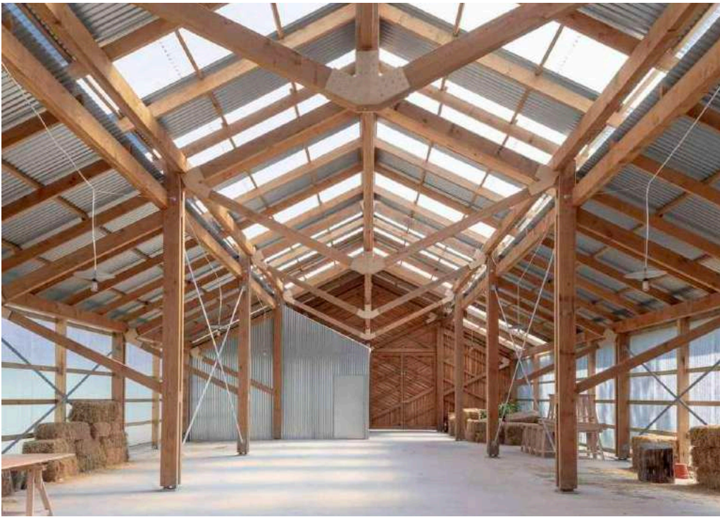
Expressed heavy timber structure, Waterloo City Farm by Feilden Fowles, London
